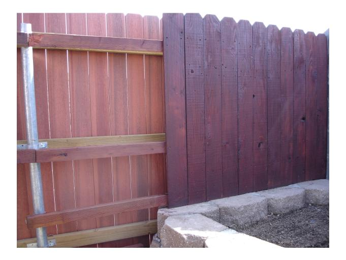
Example of compliance with the construction detail as shown on page two. Construction method uses Simpson Strong-Tie PGT2Z-R 2 3/8" Inch pipe gripe tie with attached pressure treated horizontal framing to which interior fence pickets are secured.
